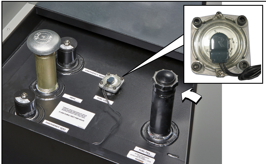
Figure 5-7. Check Fuel Level Gauge and Fill
